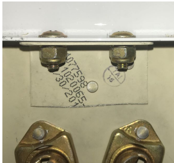
Figure 8-20 Formed Clip to C-Channel Installation
